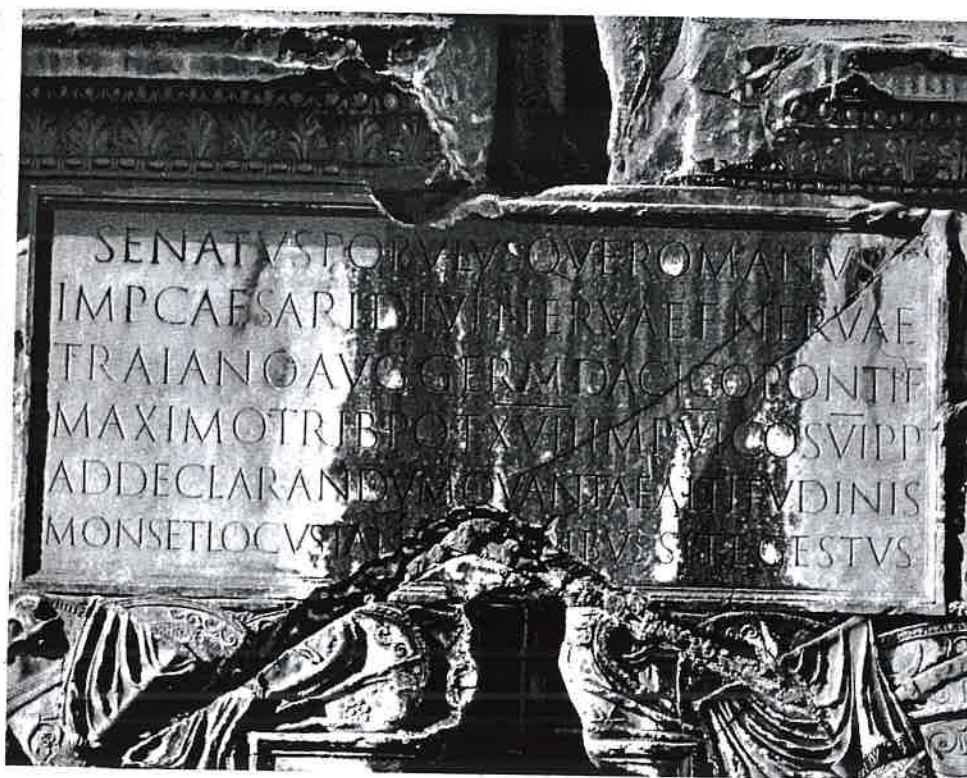
Fig. 70. A photograph taken in 1897 before the Trajan Inscription was scrubbed with acid to remove the weather staining, moss, and soil crusts caused by the broken-out section of the projecting cornice. The acid cleansing was done in the interest of the tourist trade.
