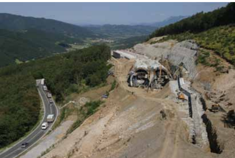
Construction of a covered pit, Rebernice
